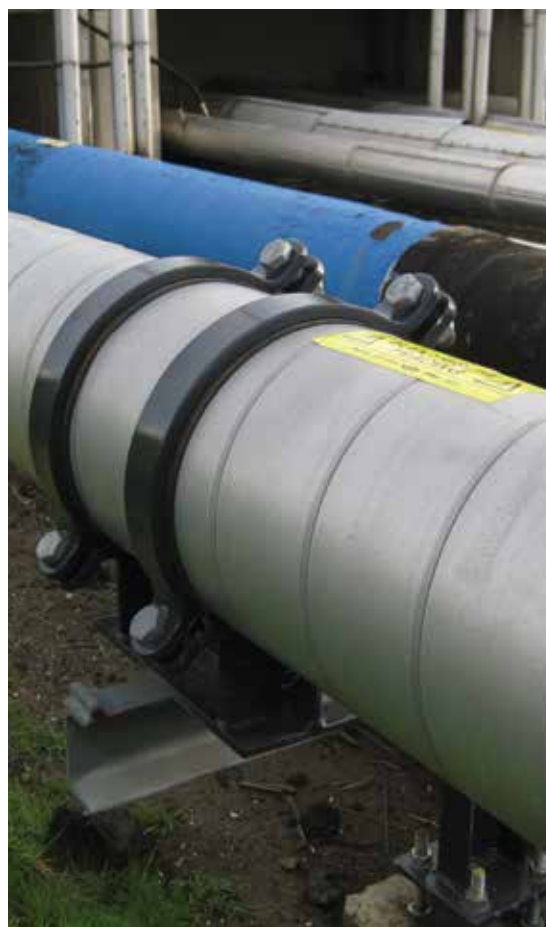
Pipe supports installed over the cladding guarantee uniform thermal profile along the entire pipe length.
